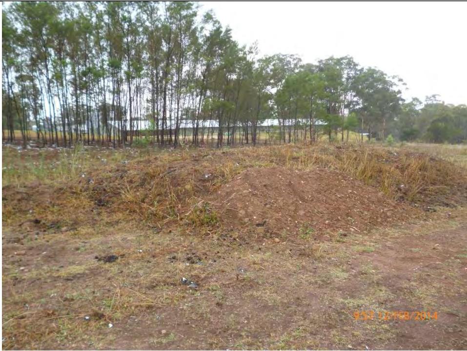
Plate 26: Fill stockpile located on Lot 6 (12/02/2014)
