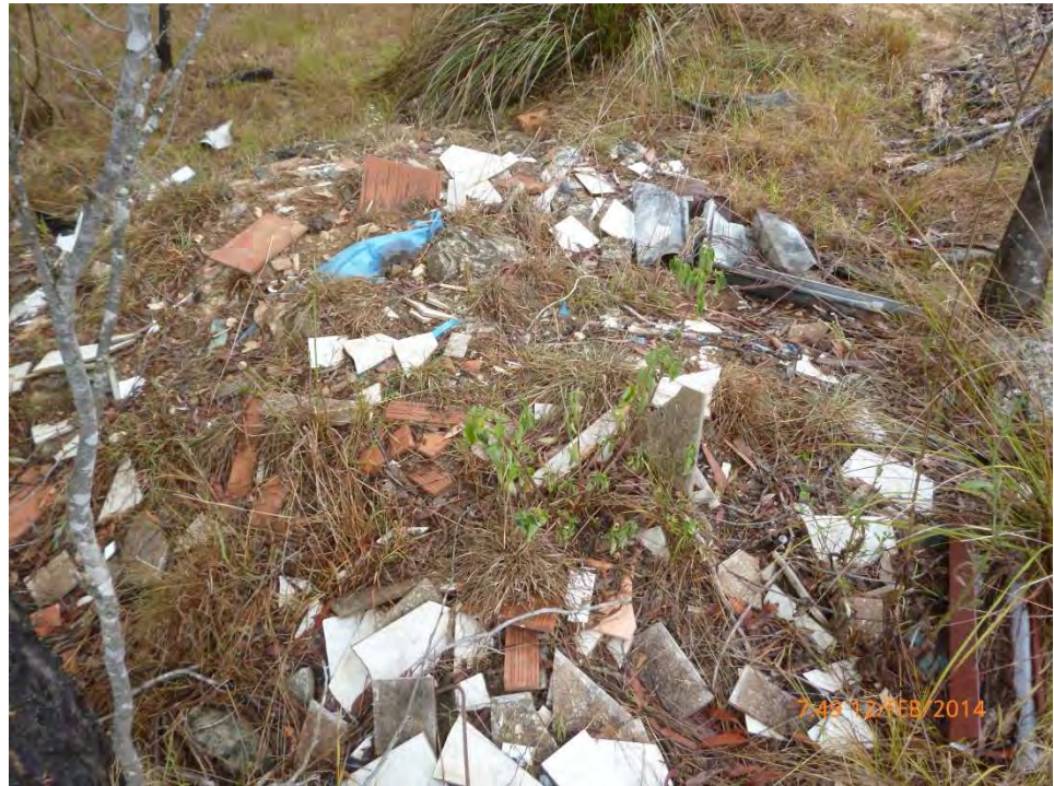
Plate 12: Fill stockpile located to the east of Lot 121 (12/02/2014)
